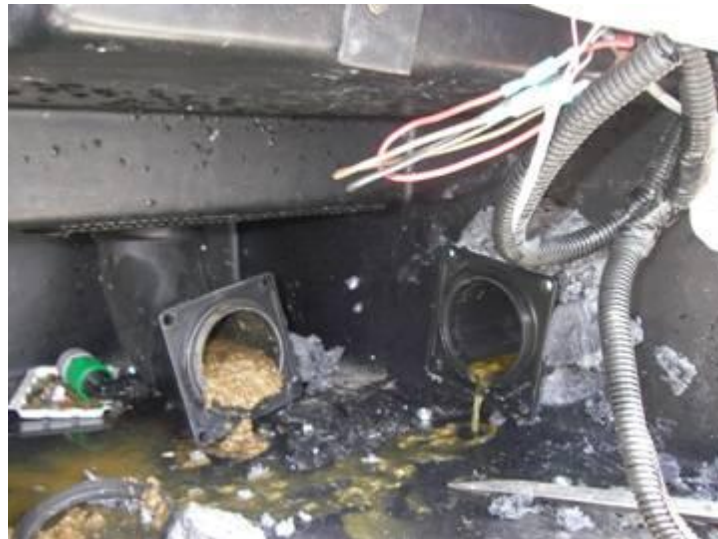
After Removing Valves and Manifold
